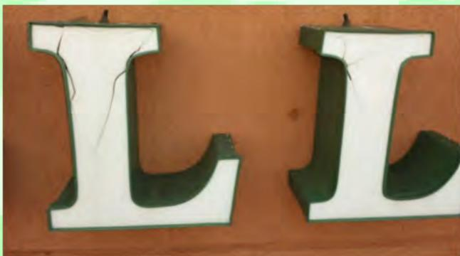
store sign. We took tracings of each of the letters and matched the plexiglass color to the available shades. Much like going to the paint store, plexiglass has a swatch test sample of colors and they need to match perfectly, not just in color, but also in transparency. You need to hold the test swatch up to lighting to make sure that the transparency is the same as that of the current plexiglass that is in the sign to make sure the match is accurate.
